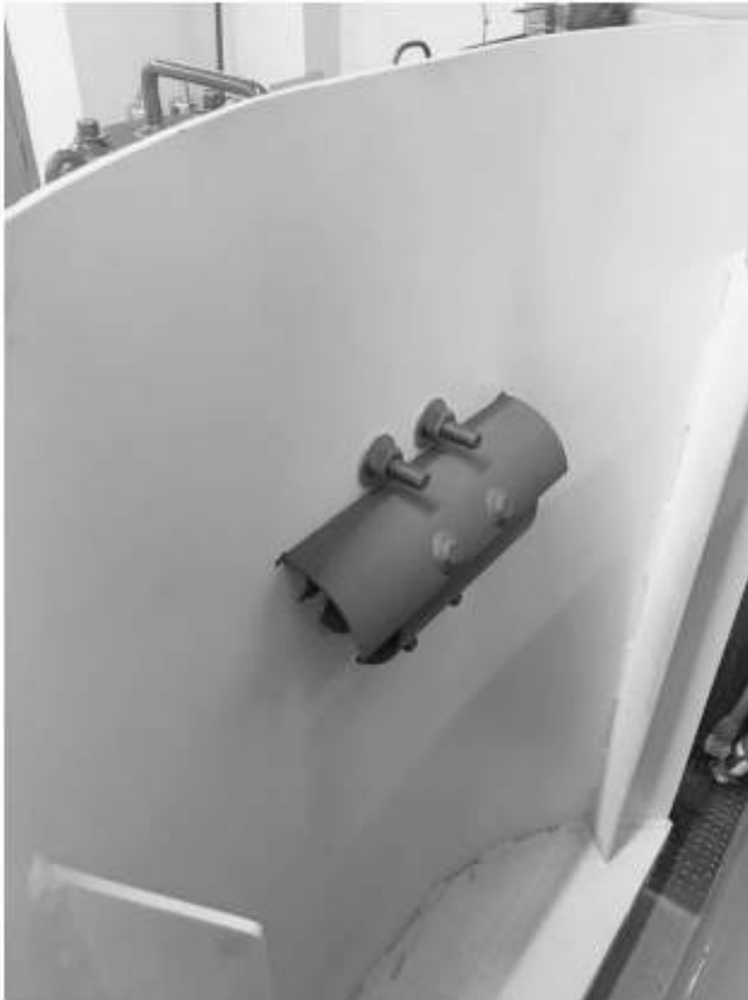
FIGURE A.5.2.5.2.1(b) Foam Chamber Deflector.
